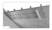
1. Fix the vapour control layer strips horizontally (preferably from top to bottom) or vertically with inscriptions on the inside with pre-installed double-sided tape (e.g. Corotop MIX) or, if the situation requires it (e.g. timber frame), with a stapler. Cover the places where the vapour control layer is perforated by staples with adhesive tape (e.g. Corotop FIX).
